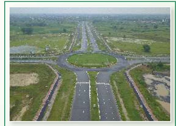
Wide roads with service lane, cycle track and pedestrian path and all utility ducts beneath
