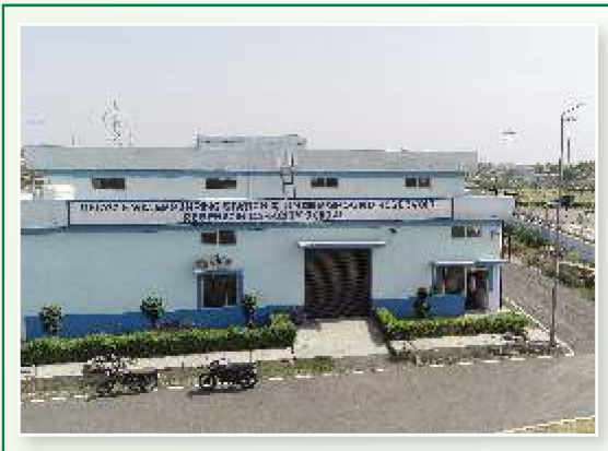
7000 kilo litre recycle water reservoir
