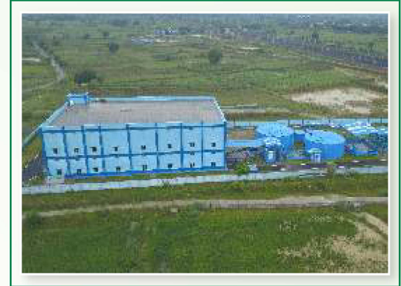
Automated Waste Collection Utility and Bio-Methanation Plant for Solid Waste Management
