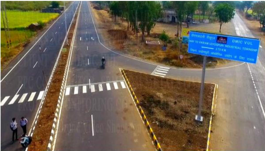
Roads and Services for Integrated Industrial Township, Vikram Udyogpuri
