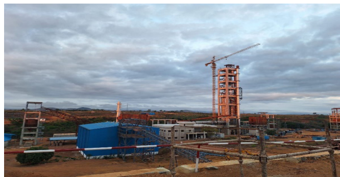
Project erection activities at site for setting up a 600 tpd cement plant in Republic of Congo
