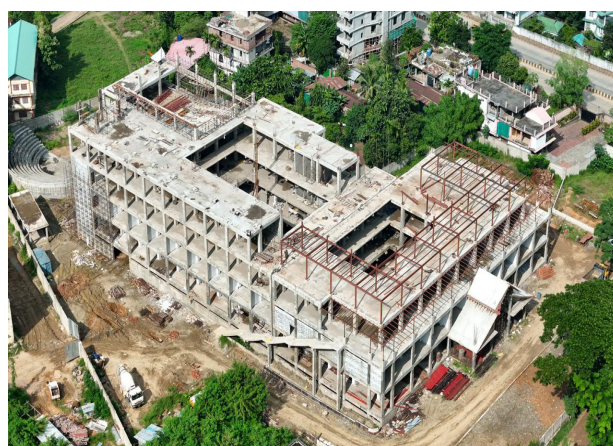
Pictures of PM Ekta mall under construction in Nagaland
