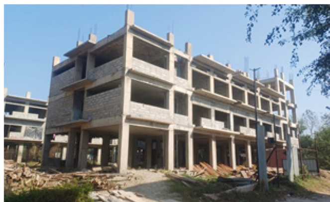
Construction of Girls Hostel at FDDI, Banur in progress
