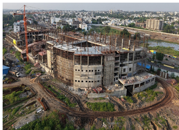
Pictures of PM Ekta mall under construction in Madhya Pradesh
