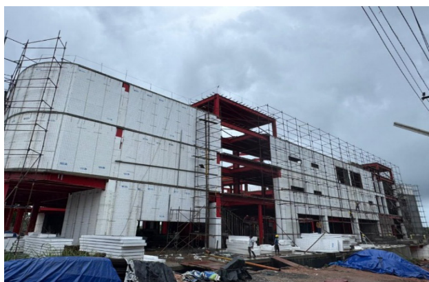
Pictures of PM Ekta mall under construction in Kerala
