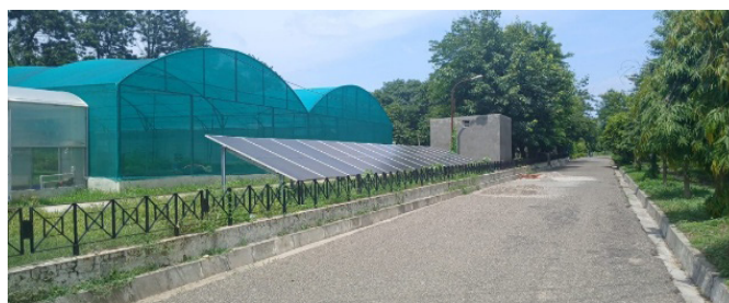
Hardening Chambers and Solar Panel
