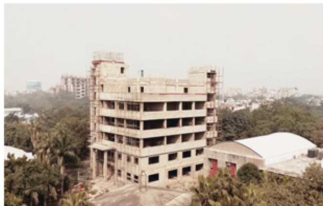
Construction of New Lab Building at FDDI, Noida in progress
